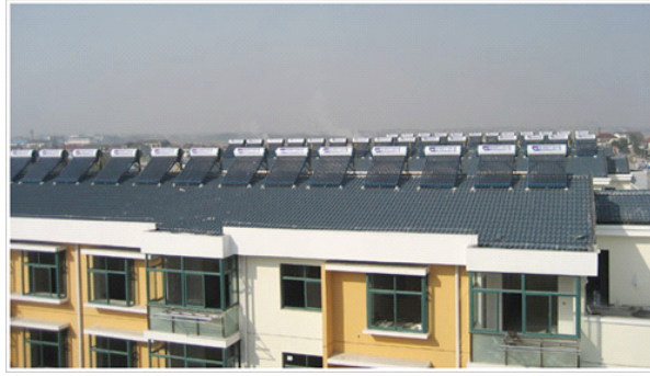
Figure 5 Solar-absorbent materials to heat bathwater
