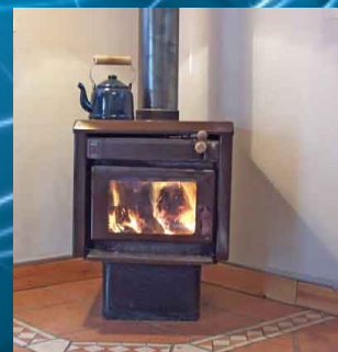
Figure 5. Typical double-chamber (slow combustion) wood-burning stove used in southern Chile. Source: http://www.aproyoestuel.com.ar/assets/images/estufa03.jpg
